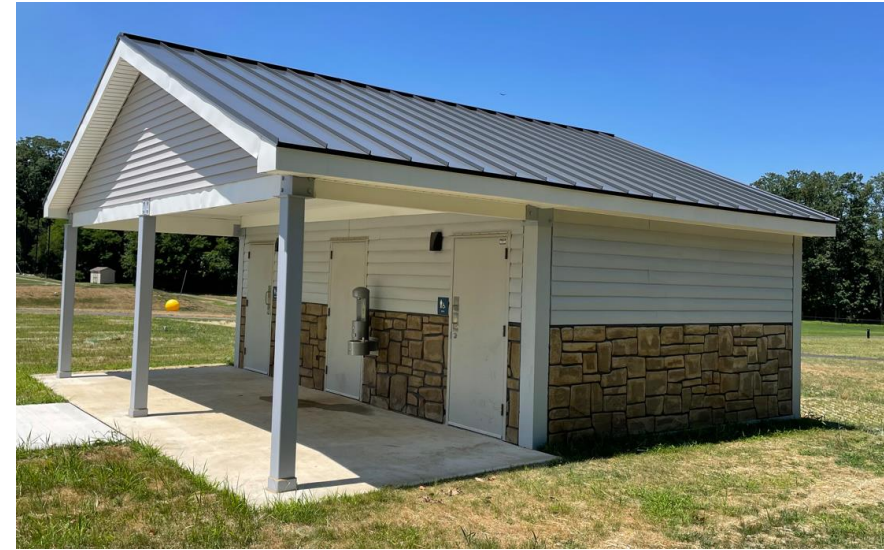
Existing Restroom Building at Sycamore Recreation Complex
