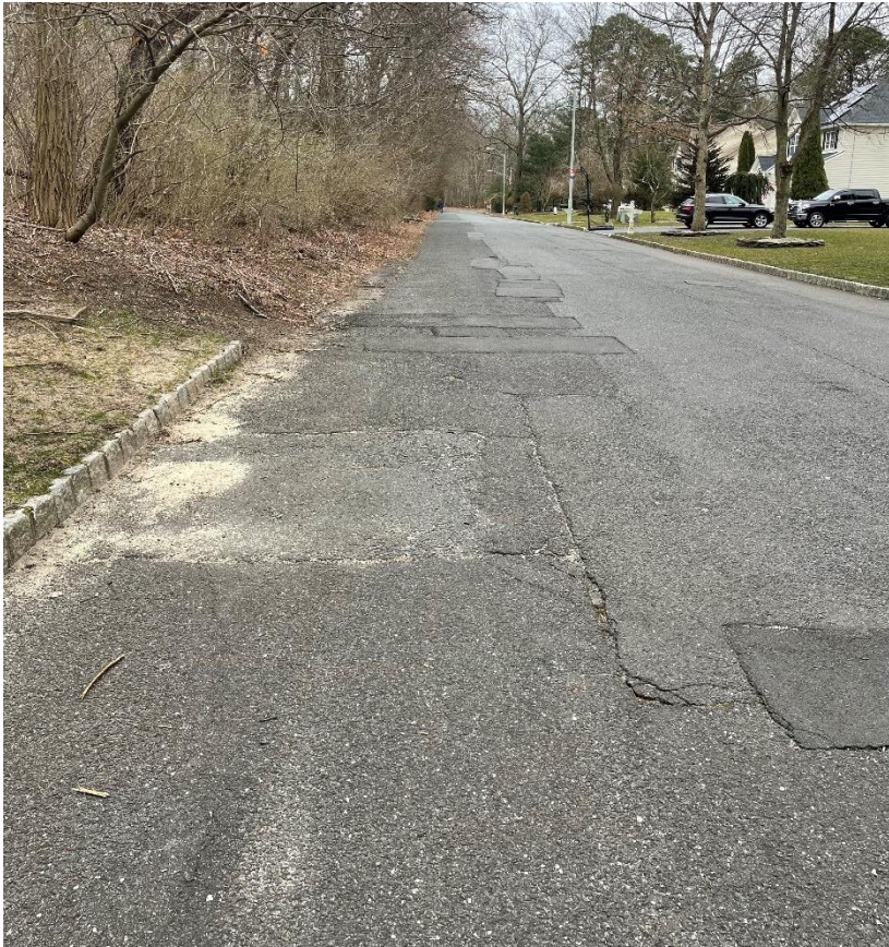
Harvard Drive Existing Conditions
