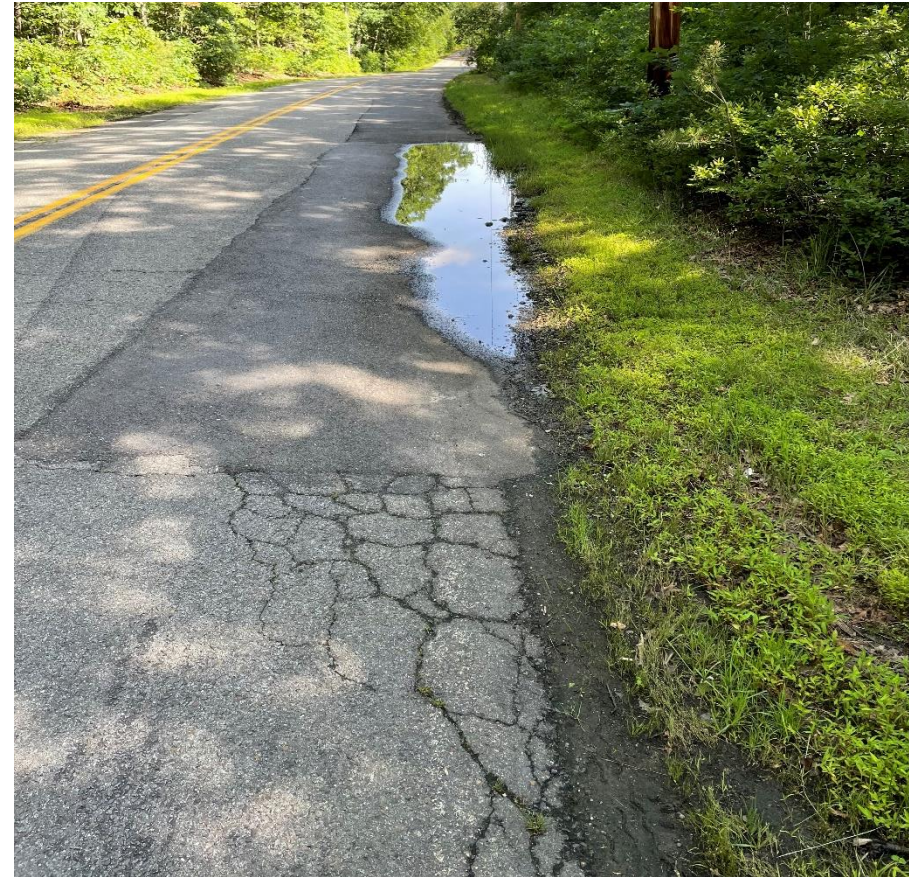
Wardell Road Existing Conditions
